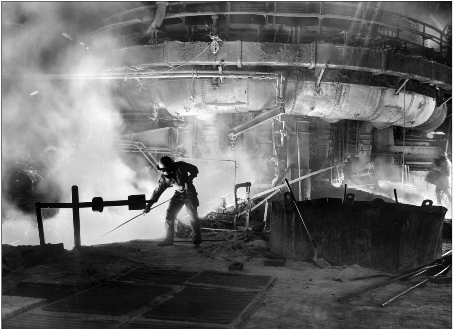
October 10, 1951 – A worker in the blast furnace at Sparrows Point (Robert F. Kniesche/Baltimore Sun)
