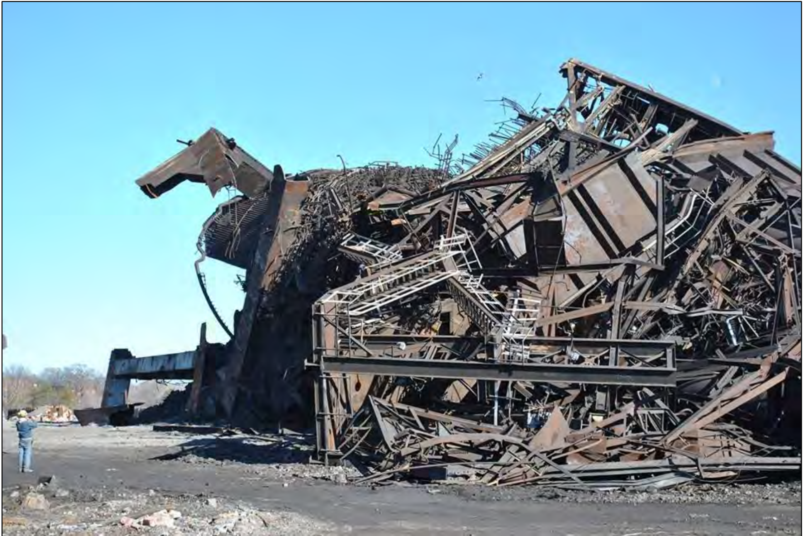
Demolition of the “L” Furnace—January 28, 2015
